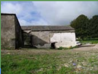
Barn 2 - raw state then complete
